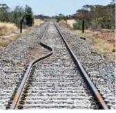
Fig 9.7 (a) Thermal expansion
