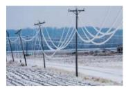
Fig 9.7 (b) Thermal expansion
